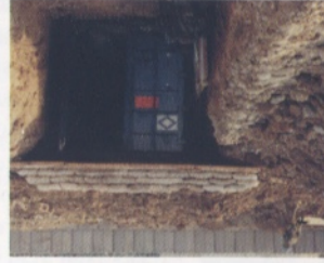
Far left: The rear gate sangan, but by mortar fire on June 6th Left: An ISO container dug-in by the Engineers to provide bomb-proof collective protection
