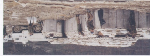
Top: The Pioneer platoon constructing bomb-proof collective protection during March and April
